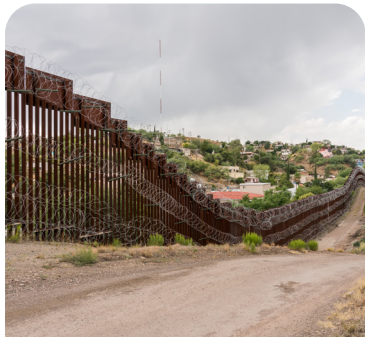
The US/Mexico border fences in Arizona, USA
